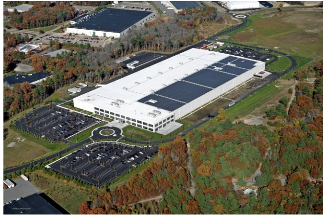
Martignetti's 680,000 sq. ft. warehouse
